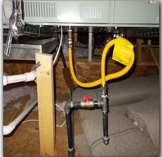
Samples of correct sediment trap installation.
