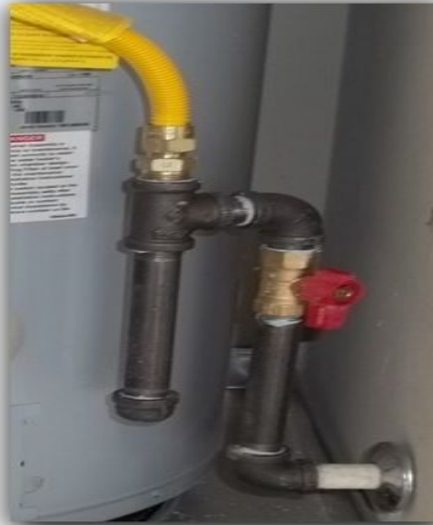
Samples of correct sediment trap installations
